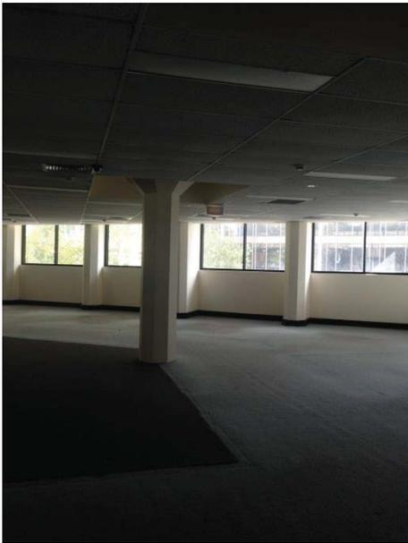
PICTURE 9 – VIEW ACROSS THE FIRST FLOOR COMMERCIAL SPACE SHOWING ORIGINAL SPLAYED COLUMNS.
