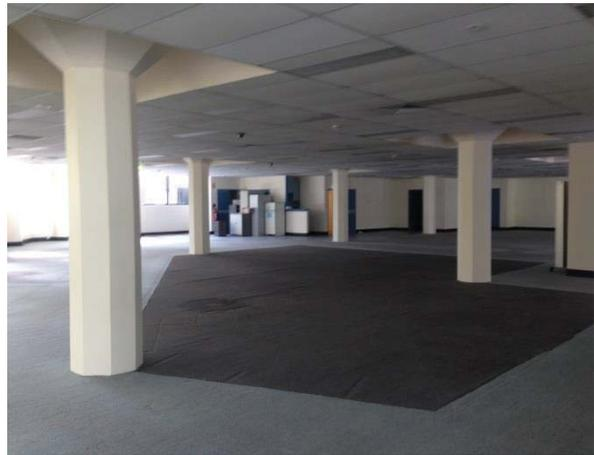
PICTURE 10 – VIEW ACROSS THE FIRST FLOOR COMMERCIAL SPACE SHOWING ORIGINAL SPLAYED COLUMNS.
